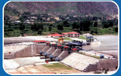
Jaypee Hydropower Plant
